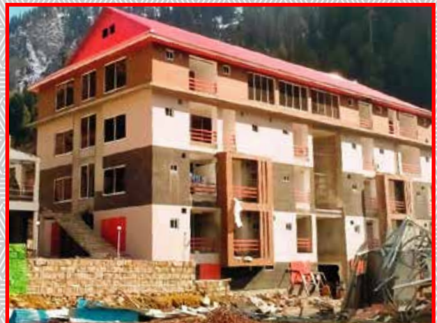
WOOD COTTAGES NARAN
